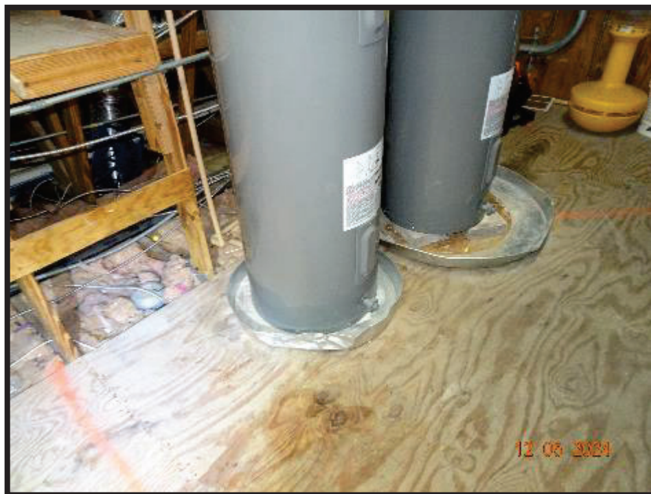
Photo 6 View of drain pans along the bottom of water tanks in the Mezzanine area. Note drain pans do not have an overflow pipe.
