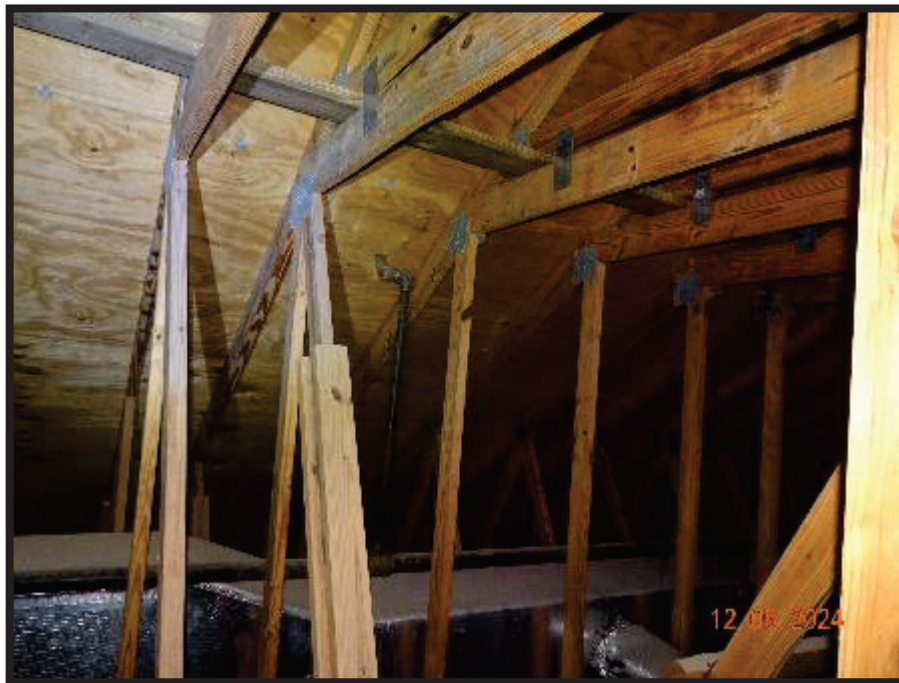
Photo 8 View of wood truss framing within the Mezzanine area. No visibly apparent evidence of water stains on the underside of the plywood sheathing to suggest moisture intrusion from the roof.
