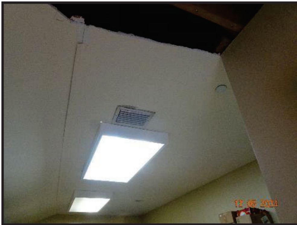
Photo 12 View of stain along ceiling diffuser along the ceiling at the entrance to the Mezzanine area.
