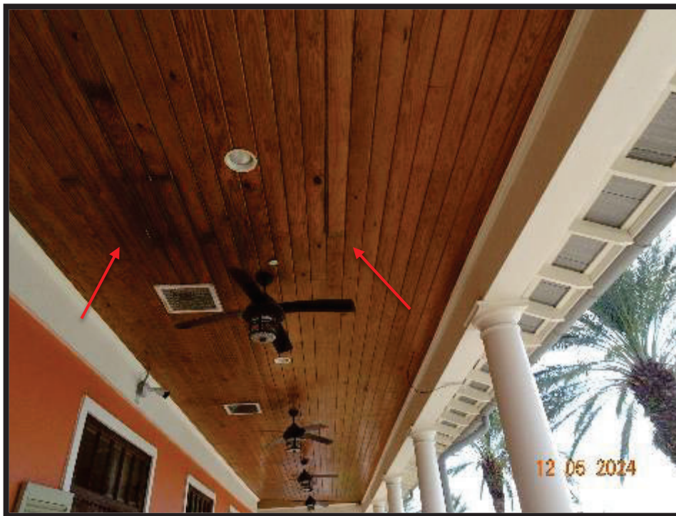
Photo 2 View of the rear patio canopy along the second floor depicting damage conditions to the wood tongue and groove planks along the ceiling.
