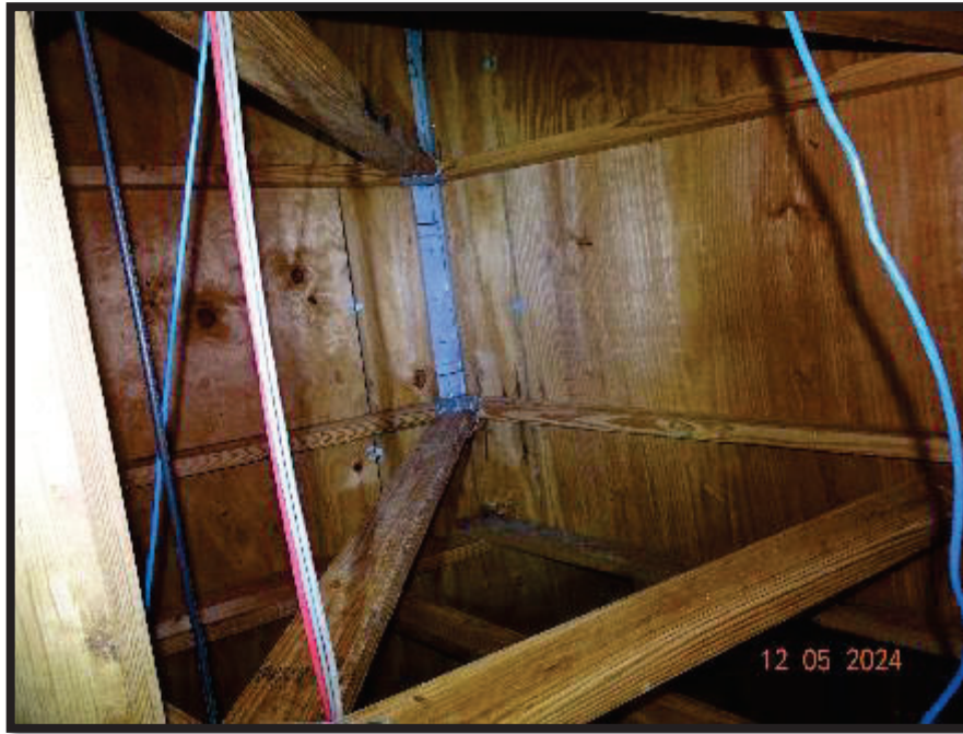
Photo 7 View of wood truss framing within the Mezzanine area. No visibly apparent evidence of water stains on the underside of the plywood sheathing to suggest moisture intrusion from the roof.
