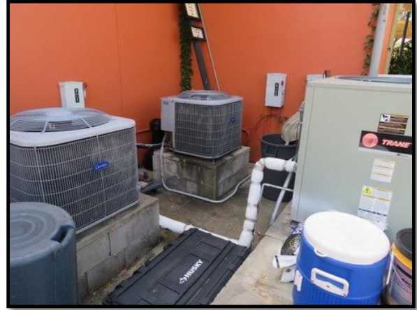
Figure 2 - Split System Condensing Units
