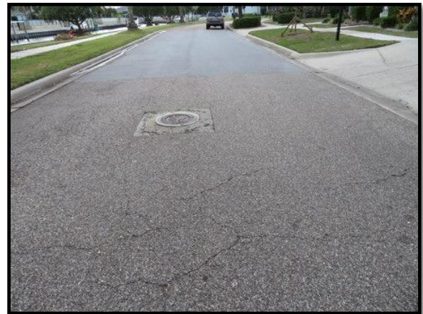
Figure 2 – Islebay Drive Cracks
