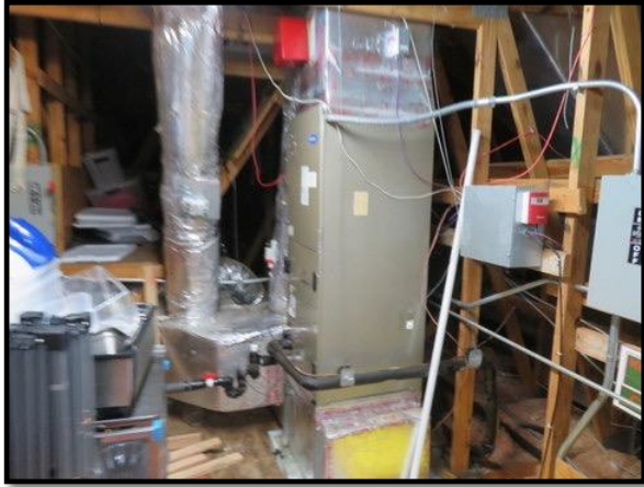
Figure 1 – Split System Air Handling Unit
