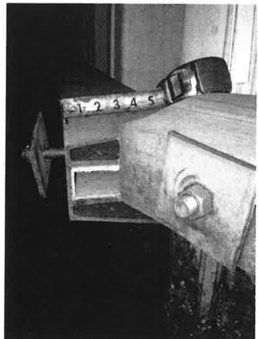
Over Stressed Anchor Connection
